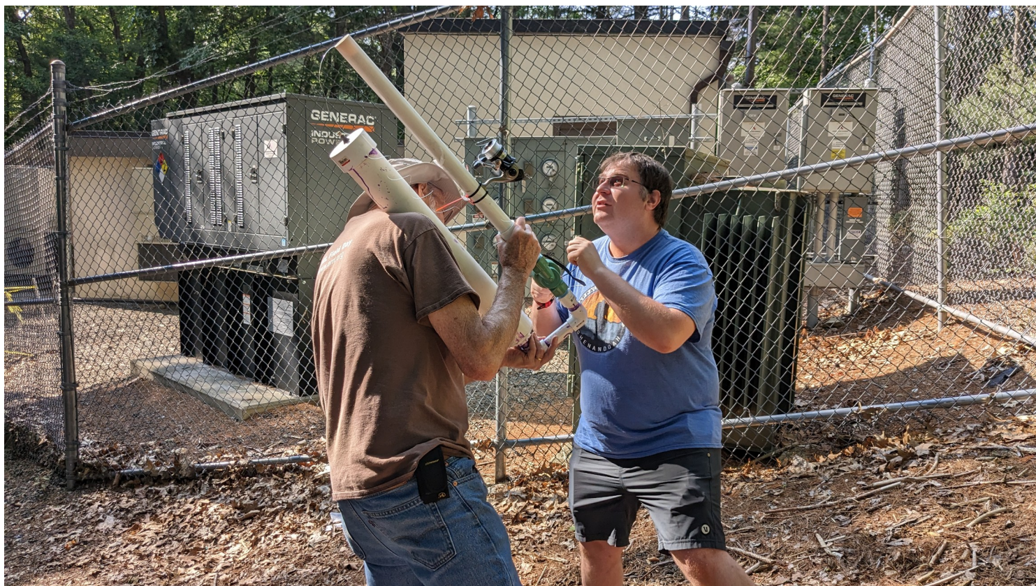
Sam W1SMF and David KB1LTW shoot lines into the trees for the future installation of our 40 meter wire antenna.
